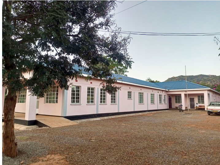
The rehabilitated Rumphu District Magistrate Court
